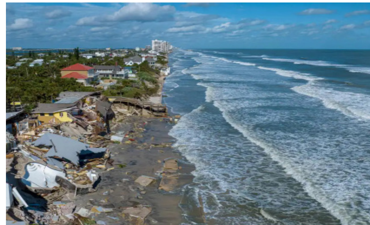
DAMAGE TO FLORIDA AFTER NICOLE LANDED ON NOVEMBER 11, 2022
